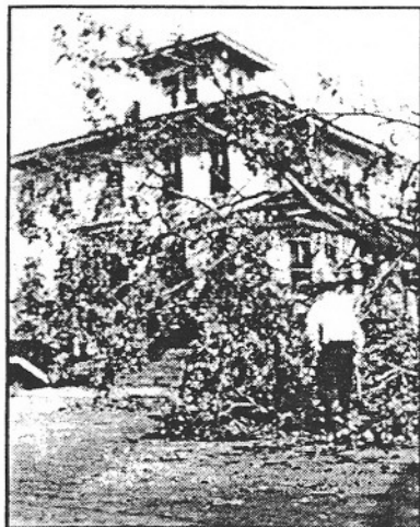
The parsonage and its elaborate cupola shown after the 1938 hurricane.
