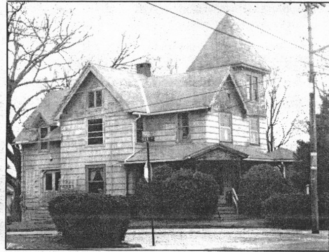
A modern-day cable TV, electric and phone lines cannot obscure Frank Larrabee's imposing Eastlake-style house, built in 1888 on the northwest corner of Prospect and Oak.
