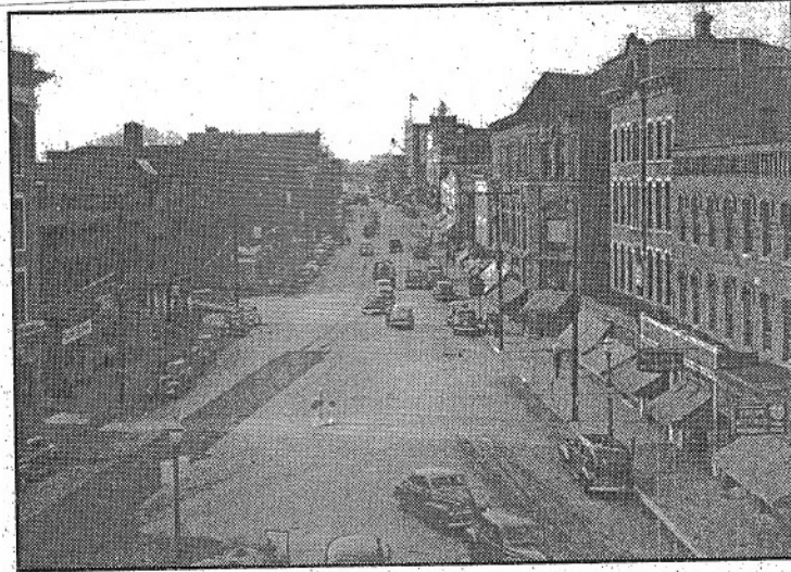
Keigwin's Commercial Block, built in 1866, was located on the north side of Lincoln Square and housed the Candy Kitchen. The Union Block stood on the south side of Lincoln Square, just west of the Willimantic Trust Co.'s building. Both blocks are visible in this 1945 photograph.
