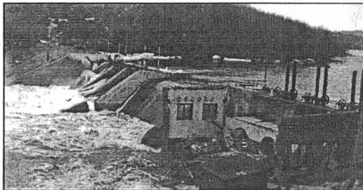
The 1955 floods caused great damage to the Scotland dam.
