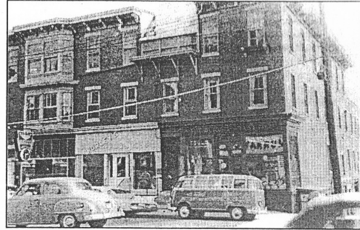
The original Hurley's store at 700 Main St. was located in the Grant-Hurley block as shown in this 1964 photograph.
