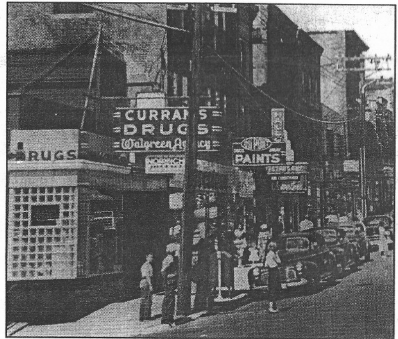
The Shea Block was partially rebuilt after the 1944 fire. It is seen here several years later in the early 1950s, still the home of Curran's Drugs store.
