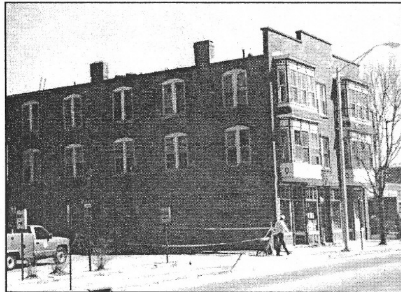
The building known as the Mazzola block was recently saved from demolition and will be renovated.
