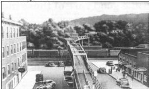
On June 22, 1906, the prefabricated sections of the bridge arrived by rail from Owego, New York, where they had been constructed in the company's workshops. It was decided to bolt the sections together on site, rather than weld them, so the bridge could be easily dismantled if the railroad companies decided it should be removed or elevated. After the sections were bolted together, the painters arrived on the scene and added coats of white, green, and black.
