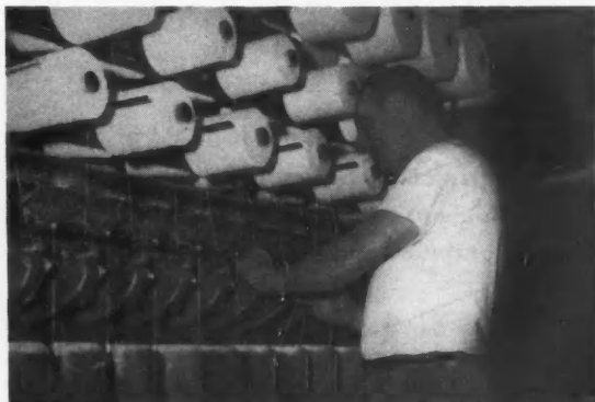
TWISTER TENDER— Turcotte tends the running of a set of twister frames in the Wool Department. His main function is to repair any breaks that occur in the yarn while it is in operation.
