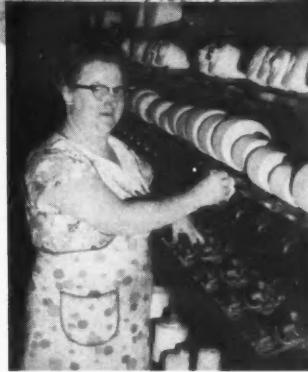
ON THE JOB —As a winder in the Shoe Thread Twisting Department, Mrs. Chasse winds supply packages for the twisters from spring supply packages from the Dye House. Roland runs the machinery that gives a glazed finish to sewing thread. It applies size and wax solutions. Heat is then used to dry these solutions or finishes. In his spare time Roland also works as a short order cook and chef at parties and wedding receptions. Both Mr. and Mrs. Chasse worked in local restaurants before joining American Thread.
