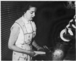
WINDER—Blanche's job involves winding single cotton yarn from spinning bobbins to wooden cones. The result is a long continuous strand of yarn used as a supply package in doubling yarn. Blanche started with the company as a learner on combers in the Carding Department, was later transferred to her present position. Isabelle started as a learner on combers—was also transferred later to the Single Winding Department as a winder.
